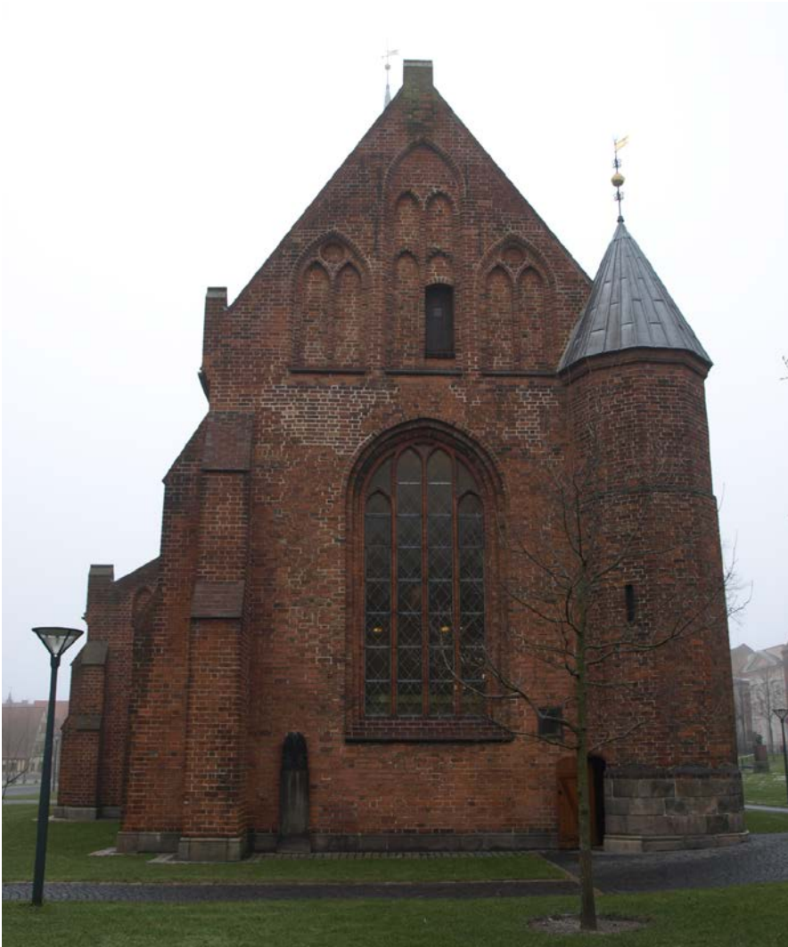
Fig. 10. The Franciscan church in Horsens. East gable. The church was heavily restored in the 19th century, however the overall phases of the buildings history are still decipherable. The east gable along with the choir was rebuilt in high gothic style during the 14th century Photo: ML 2015.
