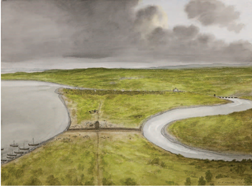
Figure 17. A reconstruction drawing of Treborgen at Ilevollene in Trondheim built around 1178–79 by Archbishop Øystein Erlendsson. A moat together with a mound and palisades cut across the mainland connecting the river Nidelva and the fjord, protecting the town from attack. Illustration: Karl Fredrik Keller (2008).
