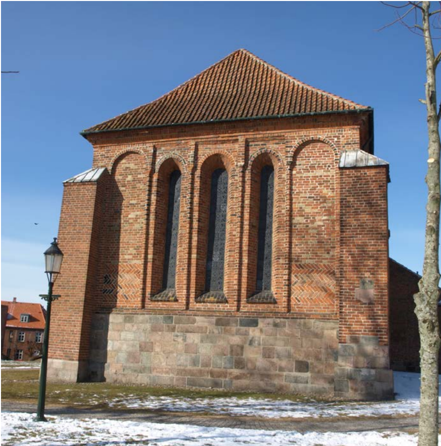
Fig. 2. The east gable of the Dominican church in Viborg. The gable was damaged by fire in 1726, after which the top was torn down – however, a detailed analysis of the gable makes it possible to partially reconstruct it. Above a granite plinth, the wall face is divided into five sections by half-columns and topped with round arches. In the three central sections, a tall, slim lancet-shaped window is placed and in the outermost sections the brickwork is laid partially in opus spicatum. Apart from the gable the façade architecture on the exterior walls with quatrefoil and circular blindings, the slim lancet-shaped windows (in some bays gathered in groups of three), and the round arched friezes terminating in pilasters, as well as the use of massive ringvaults, all give the impression of high-class architecture. Photo: ML 2014.
