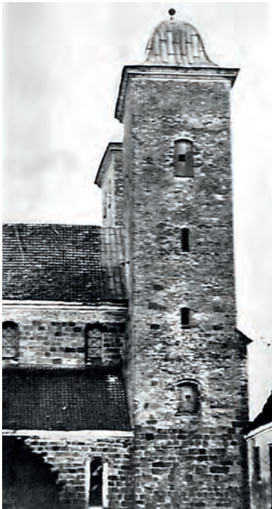
Fig. 15. Viborg Cathedral, Jutland in 1863 before restoration. The first storey of the western part in dressed stone has been heightened to towers in brickwork. Photo: Rye. (After Vellev 1976: 18.)
