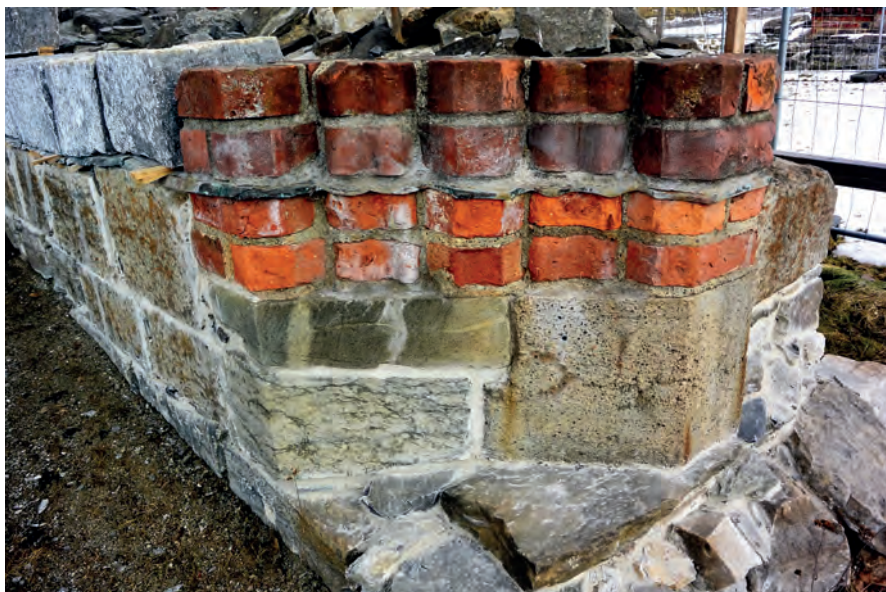
Fig. 32. The moulded splay of the west portal of the northern transept. Photo: Morten Stige.
