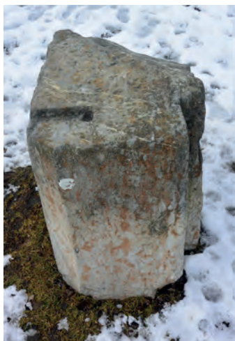
Fig. 10. The finely hewed block of orthocer limestone probably belonged to the southern jamb of the Romanesque church's west portal. Photo: Morten Stige.
