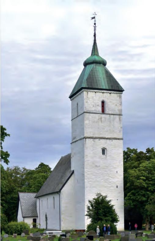
Fig. 11. Værnes church, Nord-Trøndelag is an illustration of the possible scale of the Romanesque St. Mary's and shows the imposing effect of the western tower. Photo: Morten Stige.
